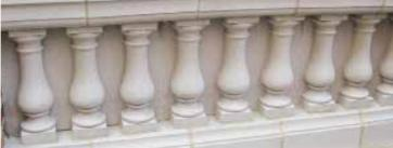
The top six stories of the eastern facade of 33 Fifth Avenue, a luxury co-op in Greenwich Village, were re-skinned as part of an exterior repair program to stop persistent leaks. The project included reconstruction of decorative stone balustrades.
