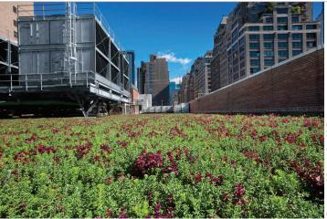
Soil and vegetation layers add insulation to the roof and protect the roofing membrane from ultraviolet radiation. They also absorb rain, reducing storm water runoff.
