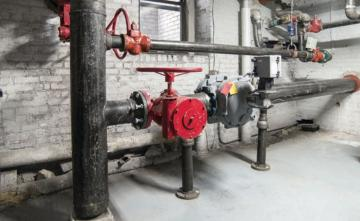
RAND designed and administered a heating plant upgrade, oil-to-gas conversion, and new chimney liner installation at 771 West End Avenue. New boiler (right, top) and gas meter rig piping (right, bottom).
