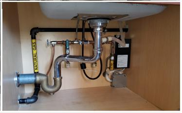
RAND's complete upgrade of the gas piping system at Belvedere East and West included (clockwise from top right): the installation of twin-set master meters, a new gas main throughout the cellar, and new gas branch piping running through kitchen cabinetry.
