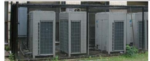
High-efficiency HVAC condenser units installed outside the building increased the library's heating and cooling capacity.
