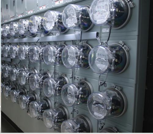
The electrical upgrade that RAND administered at Clinton Hill Apartments covered all 1,229 units throughout the 12-building complex. Newly installed equipment included submetering banks for individual apartments.
