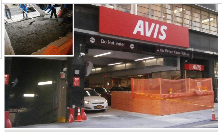
Persistent leaks in the parking garage led to extensive water damage, including badly deteriorated concrete and steel reinforcement. The repair work (inset) was phased so the vehicle rental facility could operate without interruption.
