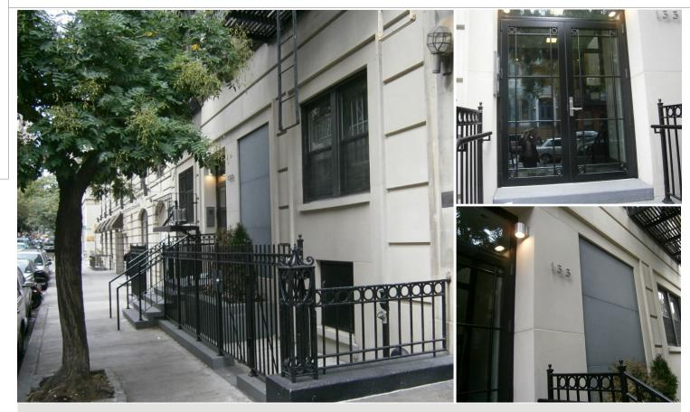
The facade beautification project at 133 East 30th Street in Manhattan included new steel fence, gate, and railing assemblies, metal and glass entrance doors, and decorative bluestone panels and curb installed along the southern facade.
