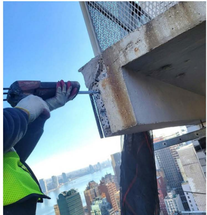
Deteriorated concrete was removed to sound substrate at the main-roof bulkhead as part of the localized concrete repair work.
