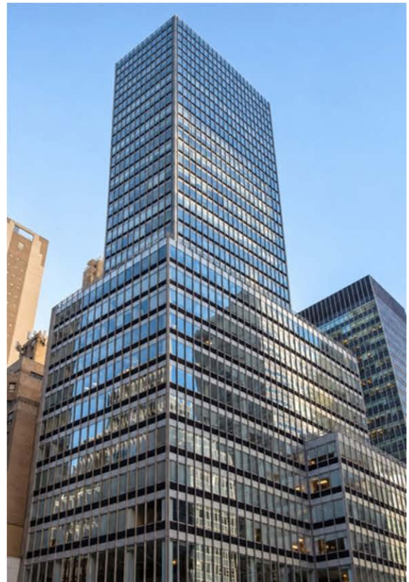
The 39-story Class A office tower is primarily clad in glass curtain wall assemblies.
