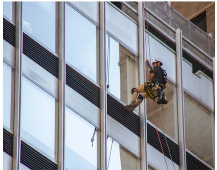
A member of RAND's in-house rope access team conducts a close-up FISP examination of the tower's glass curtain wall.
